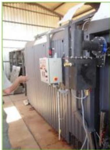
Figure 10 Stationary retort kiln (Temmermann 2016)
